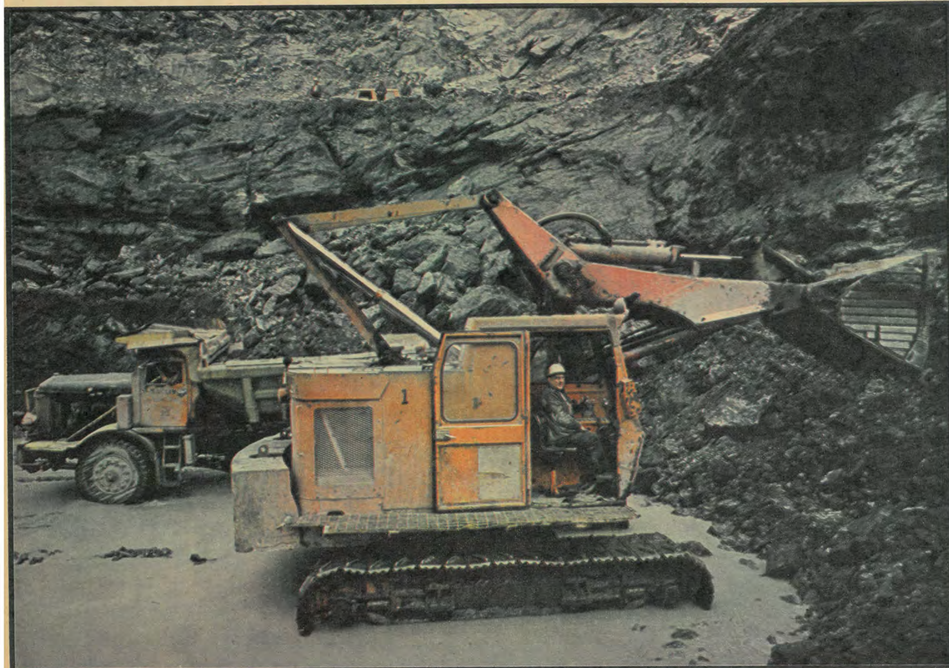
Top: Charlie Taylor, manager of Cornwall, Grace and Marmora mines, surveys the open pit operation which took 100 years of carving to create. Cornwall is where his career started.
